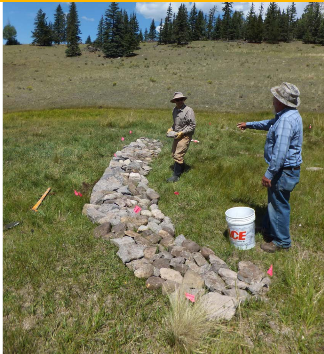
Workshops are a good way to teach volunteers how to build rock media lunas that spread water. Image credit: Karen Menetrey, Rio Grande Return.
