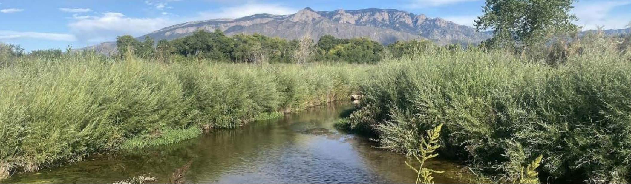
Harvey Jones Bioswale, a green stormwater infrastructure feature that provides wildlife habitat and slows stormwater and treated wastewater before it enters the Rio Grande in Corrales. Image credit: Todd Lopez, Rio Grande Return.
