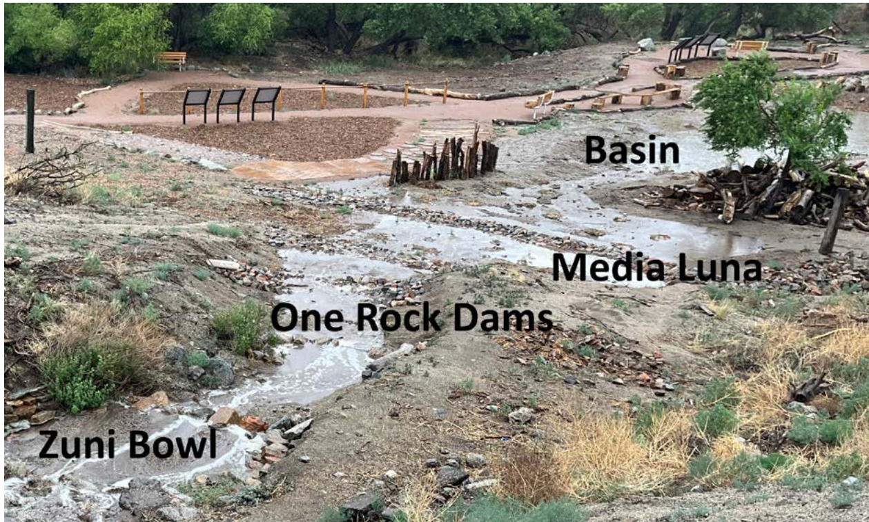
A variety of green stormwater infrastructure techniques to reduce erosion and protect recreation infrastructure at the Tijeras Creek BioZone Open Space. Image credit: Bobby Mullin, Bernalillo County.
