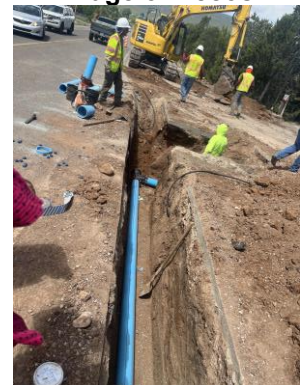
Figure 10. Waterline Replacement in the Village of Pecos.
