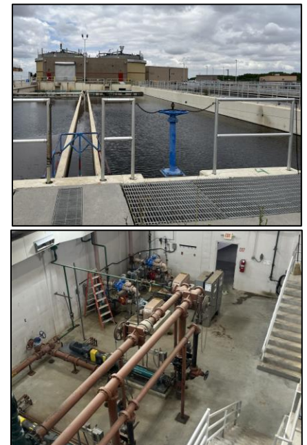
Figure 7. City of Santa Fe Wastewater Treatment Plant
